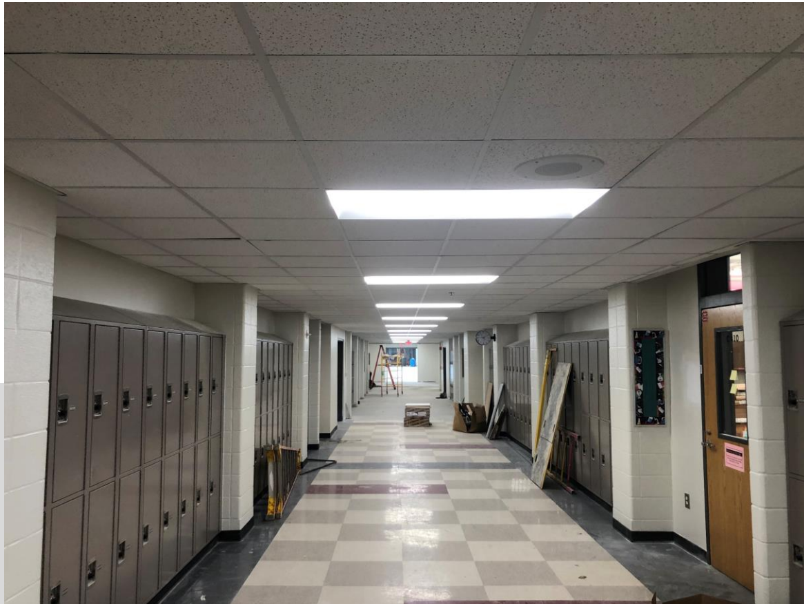
ACT Ceiling and Lights Installed in C. Allen Building
