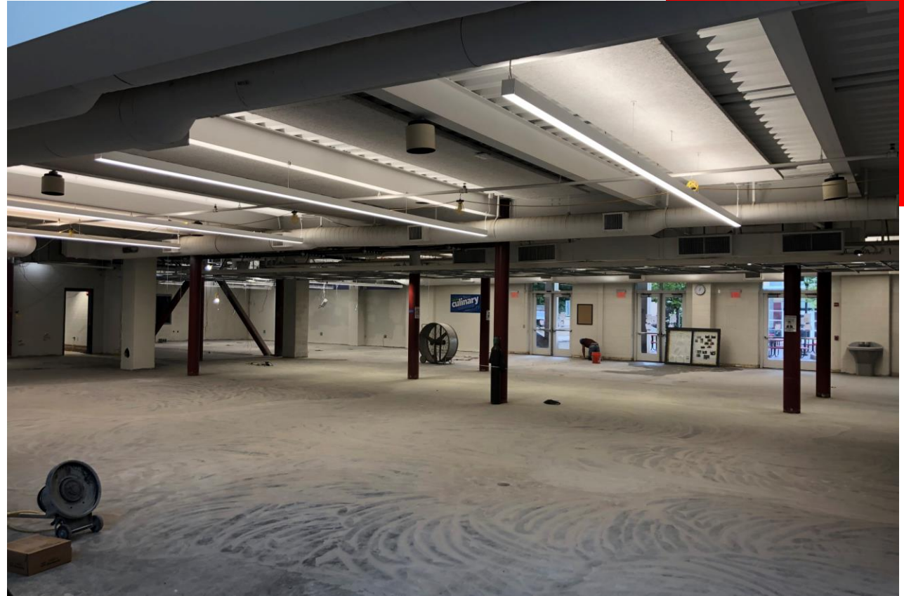
8 th Street Building Ground Floor Preparation for VCT
